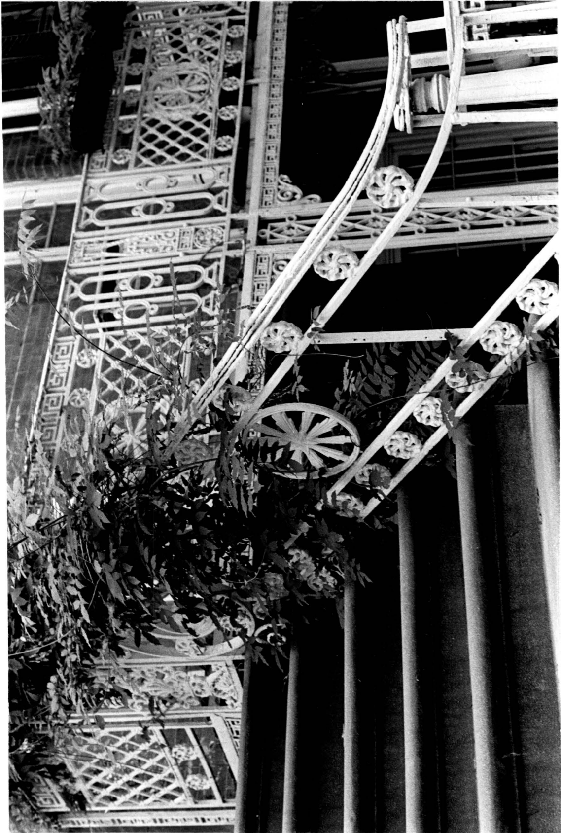
23 West 16th Street Building (ironwork detail) Photo Credit: Kevin McHugh
