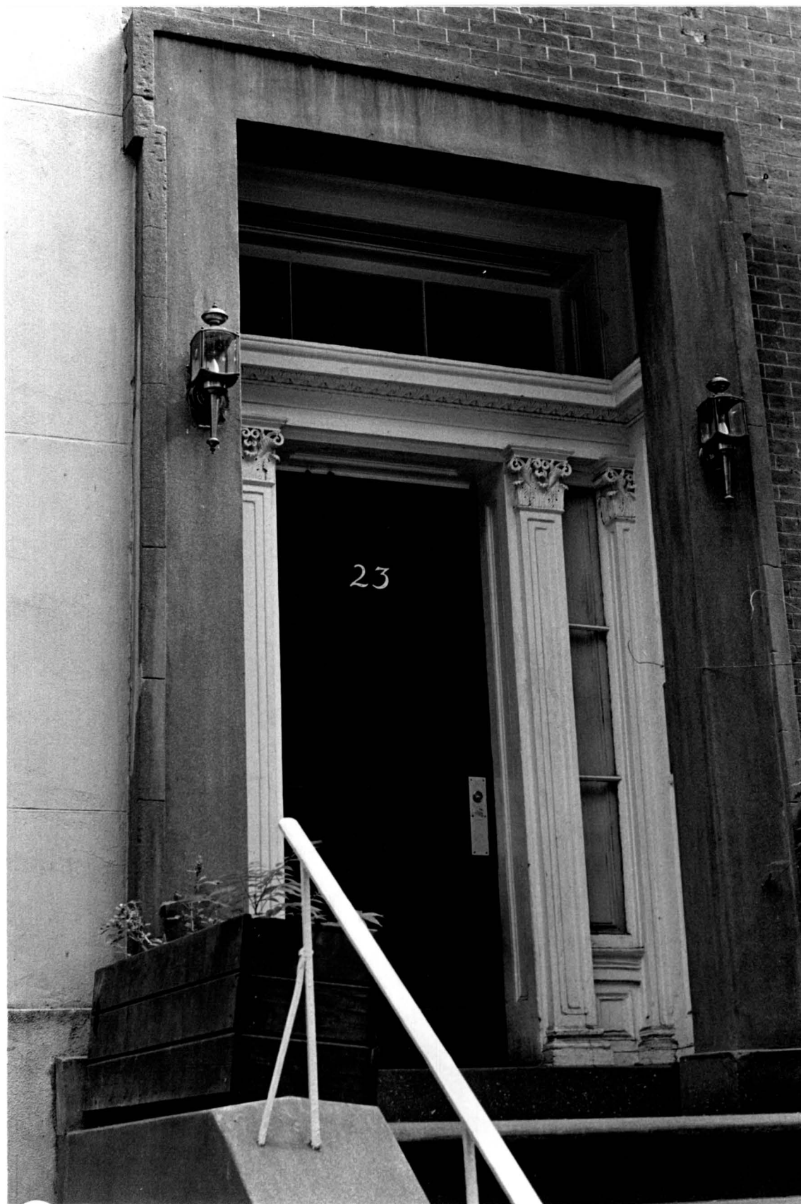
23 West 16th Street Building (entrance detail) Photo Credit: Kevin McHugh
