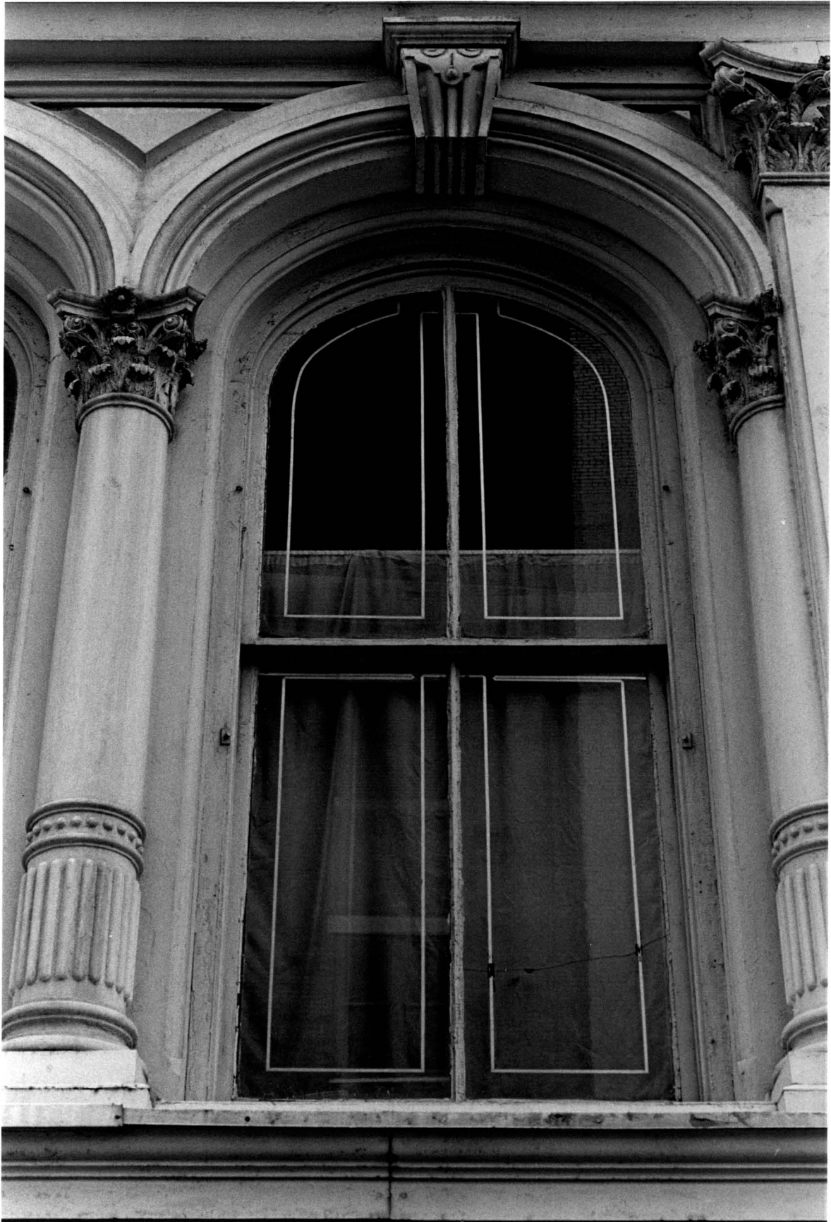
No. 319 Broadway Building Window detail, Thomas Street facade
