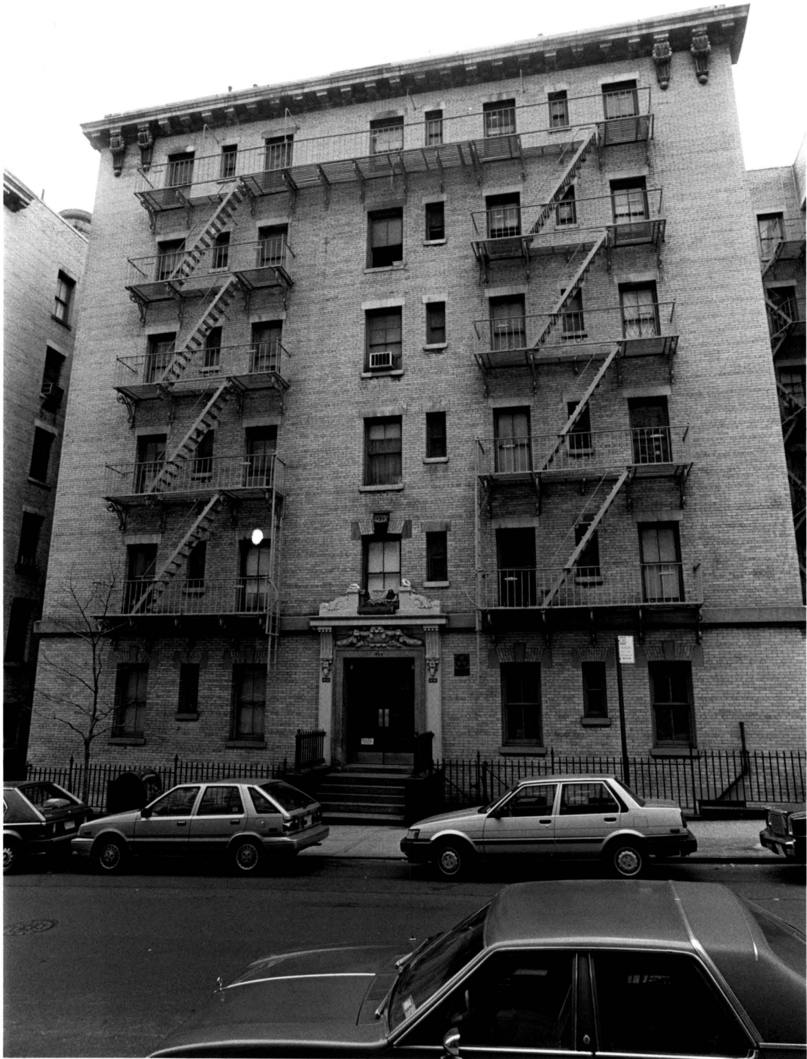
City and Suburban Homes Company, First Avenue Estate: 414 East 65 Street Photo Credit: Carl Forster
