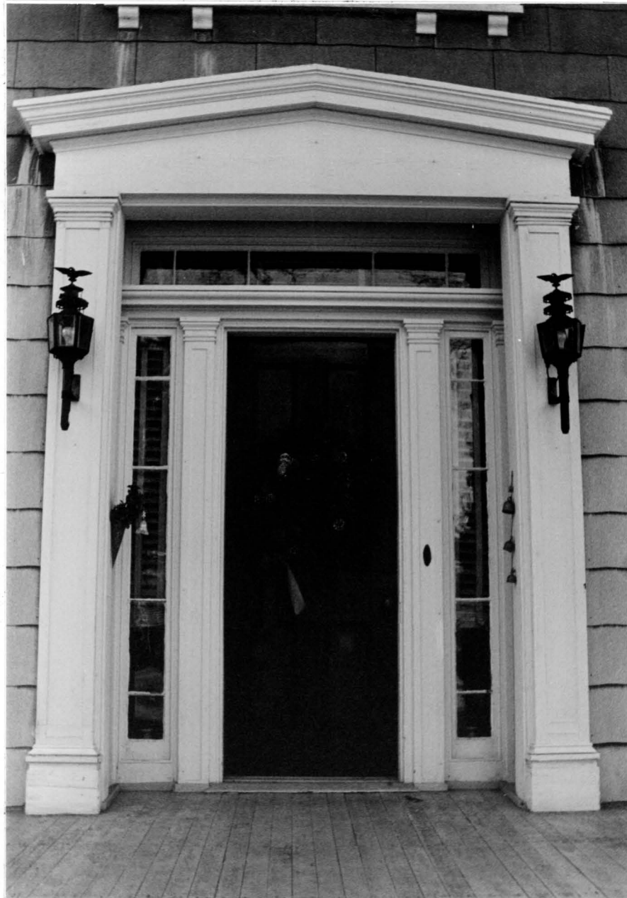
HENRY HOGG BIDDLE HOUSE, c. 1850 doorway: east elevation
