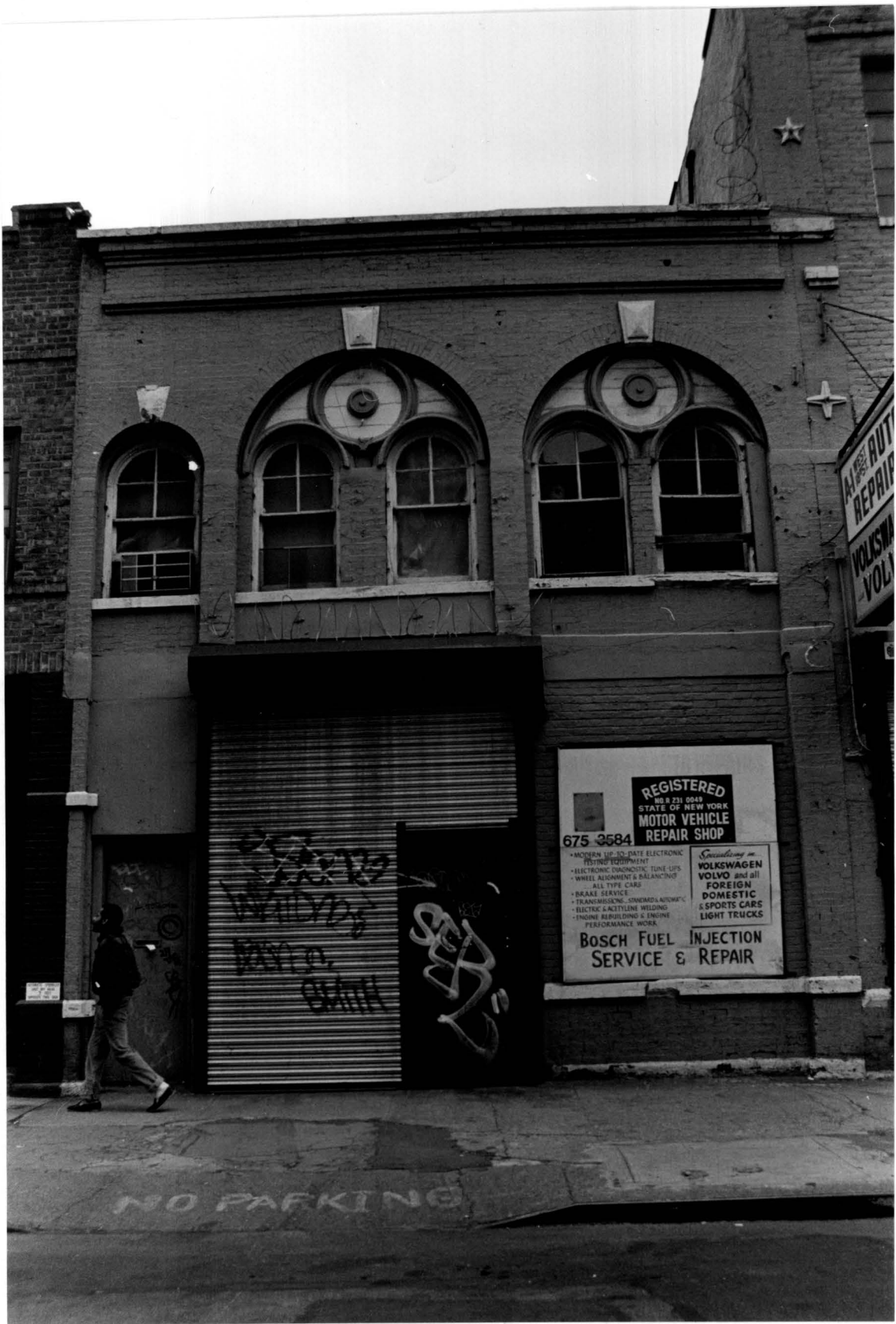
140 West 18th Street Stable, 140 West 18th Street (1865-66) Photo Credit: Gale Harris
