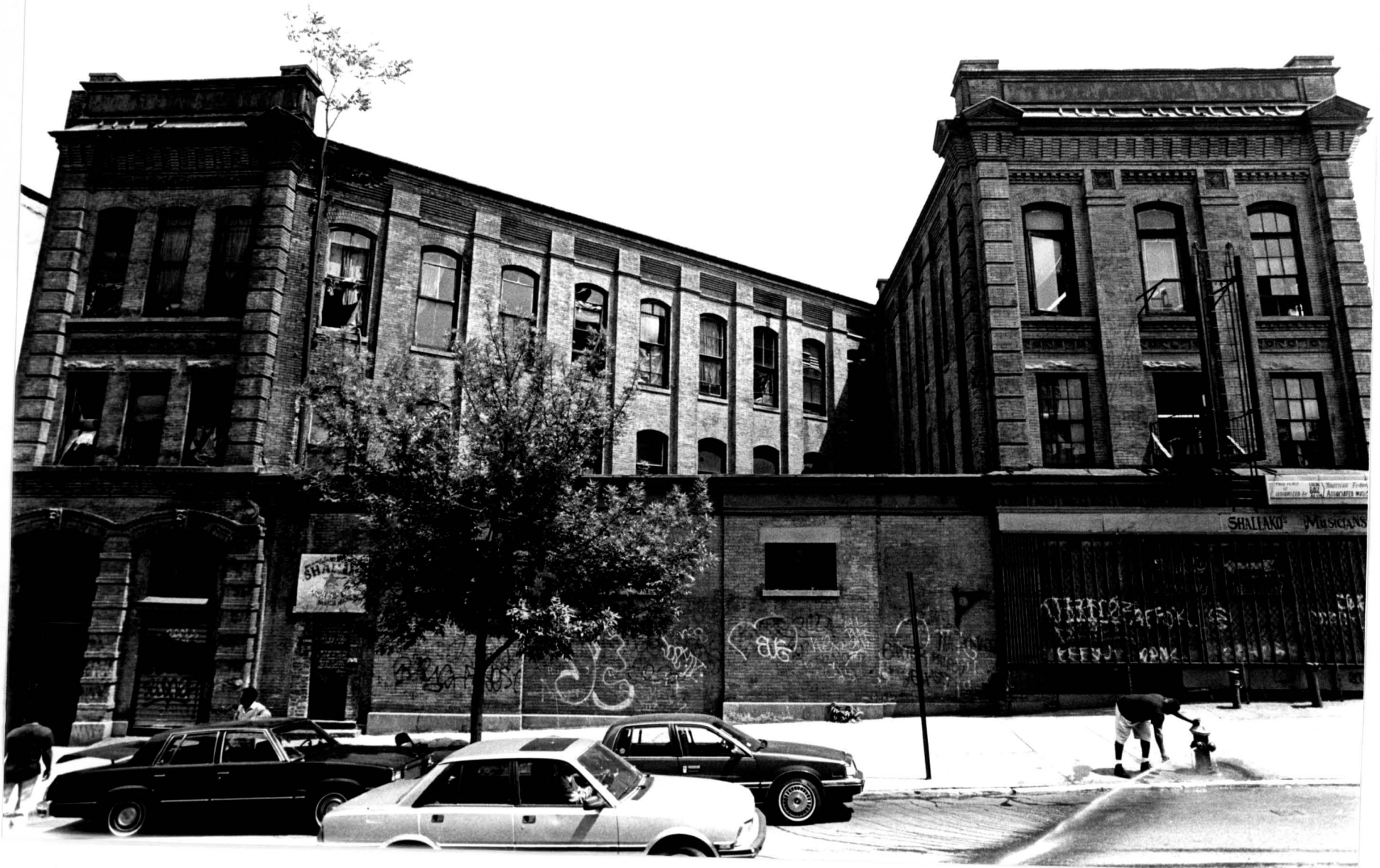
Figure 6. Joseph Loth & Company Silk Ribbon Mill, 1818-1838 Amsterdam Avenue. West 150th Street facade.
