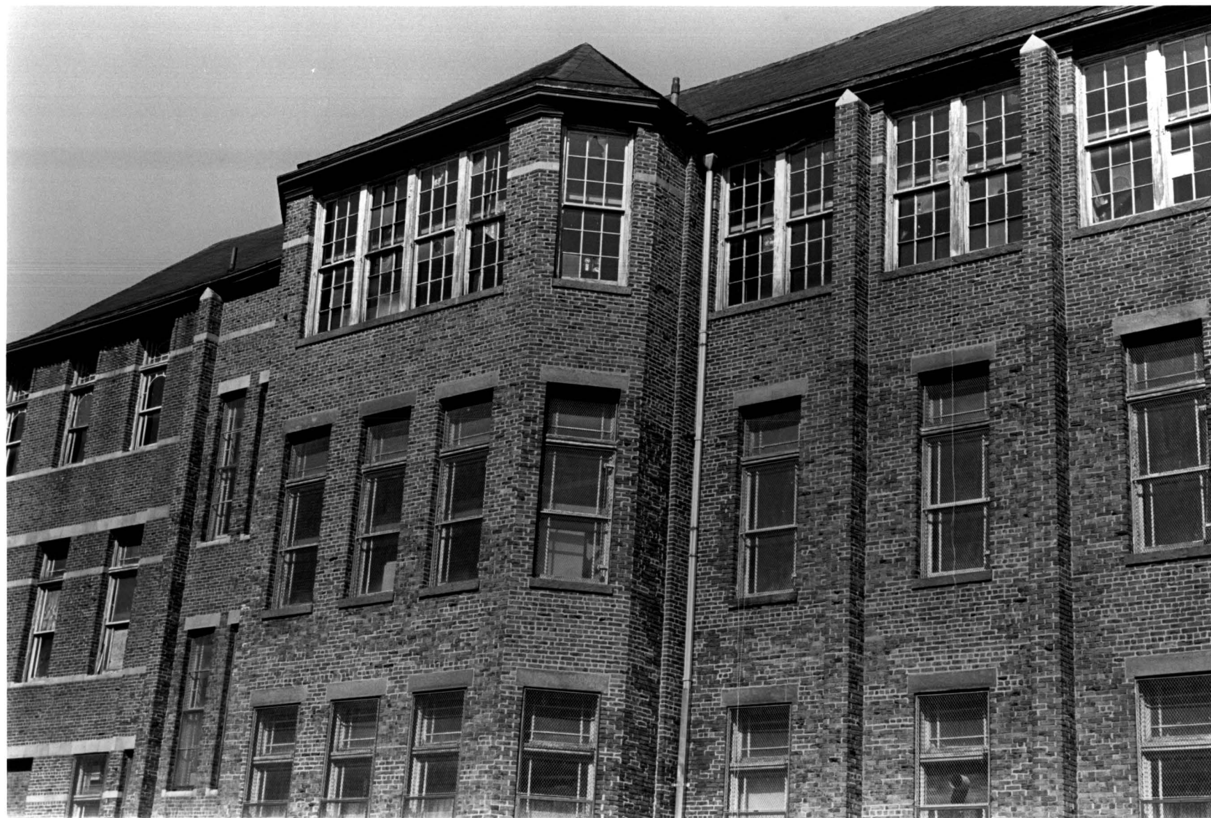
Public School 15, south facade Photo: Shockley, LPC
