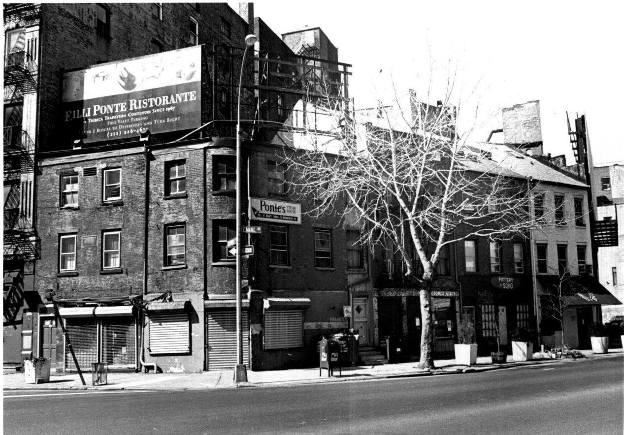
480 Greenwich Street (aka 502 Canal Street), 504, 506, and 508 Canal Street, Manhattan Photos by: Carl Forster, 1998
