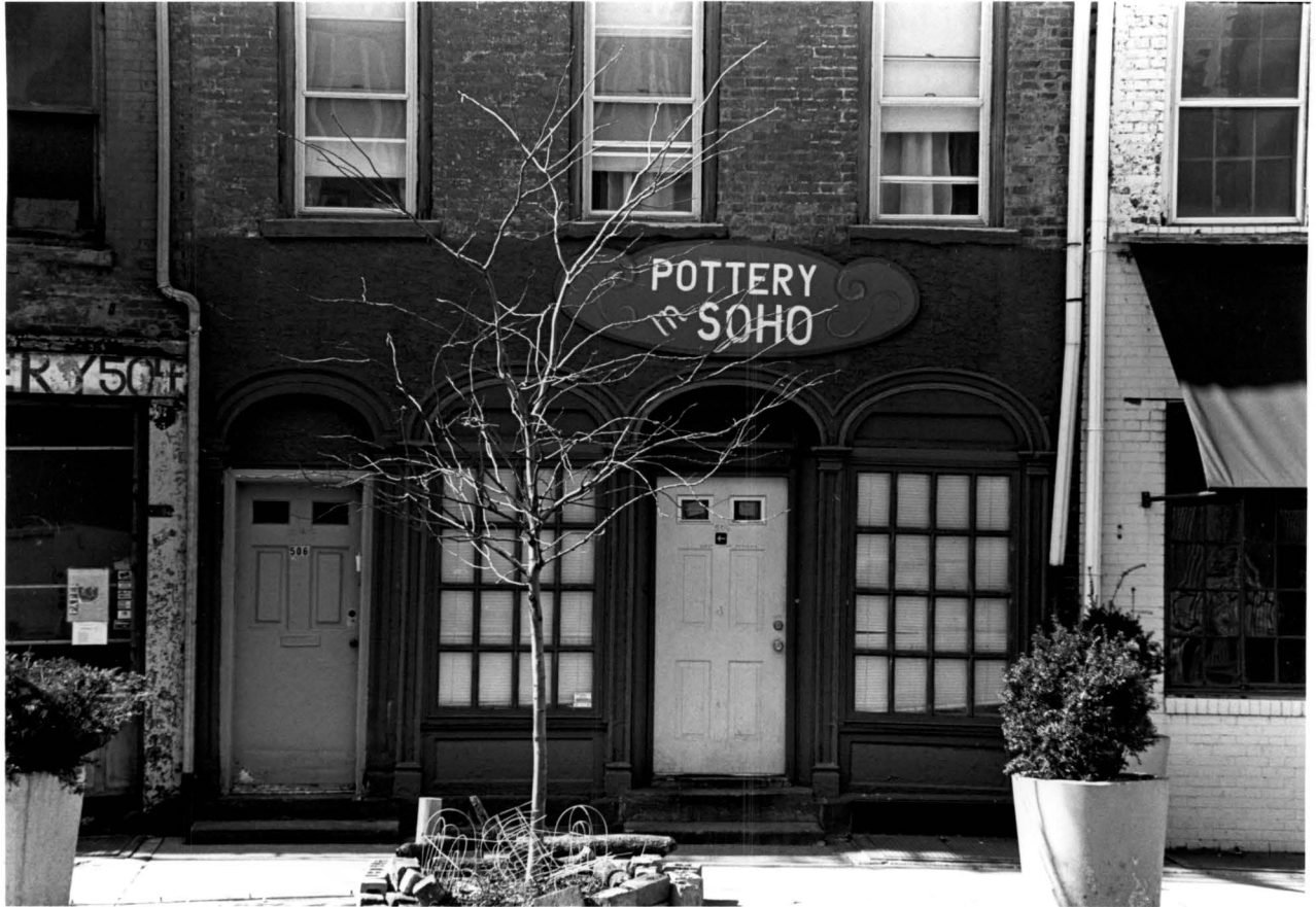
506 Canal Street House, Manhattan Storefront details
