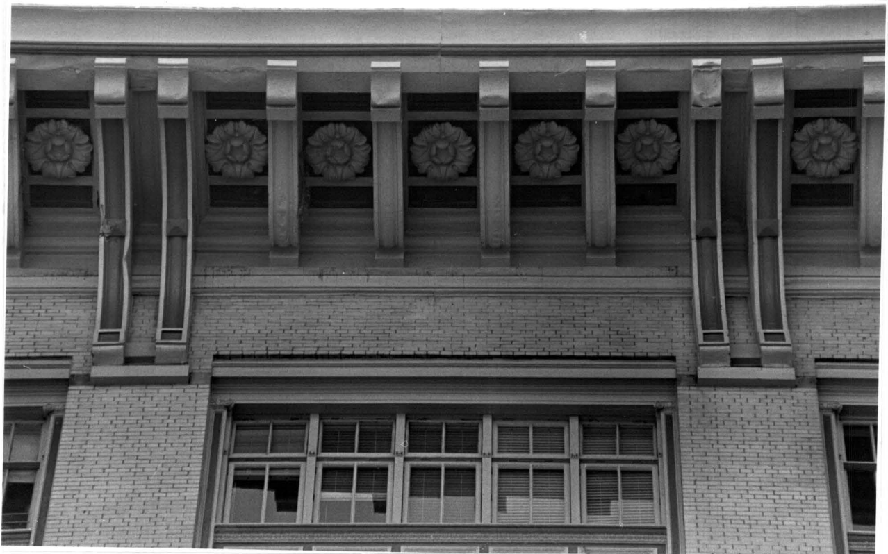
No. 130 West 57 th Street Studio Building Cornice Detail
