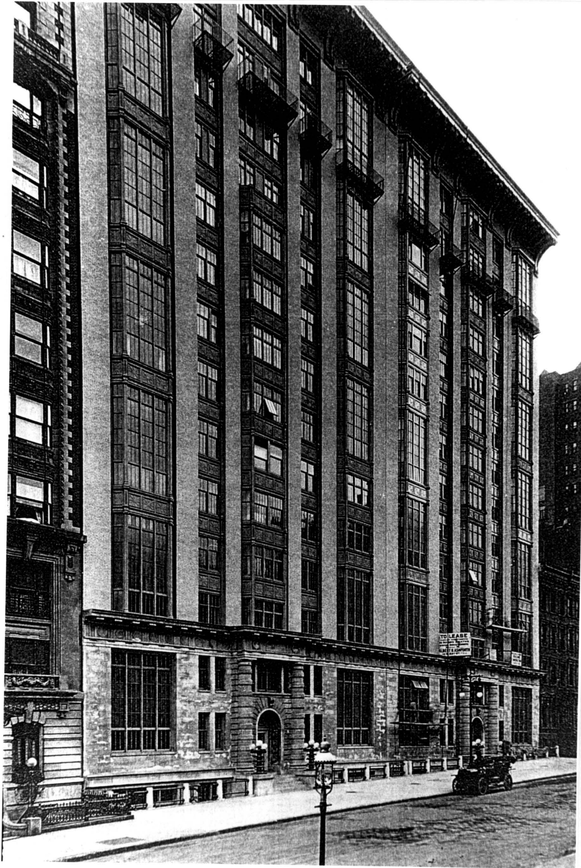
Nos. 130 and 140 West Fifty-Seventh Street Studio Buildings Borough of Manhattan
