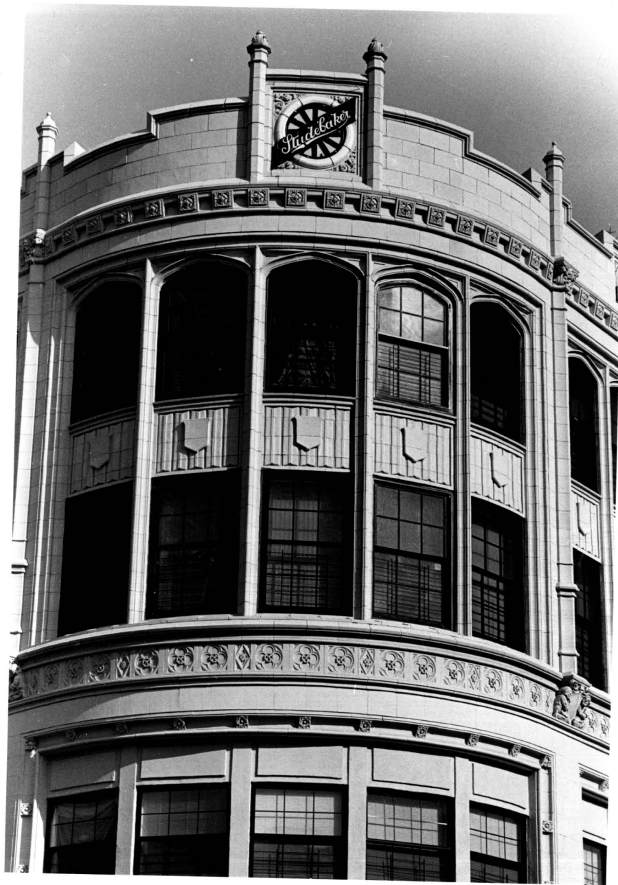
Studebaker Building, detail of corner Photo: Carl Forster
