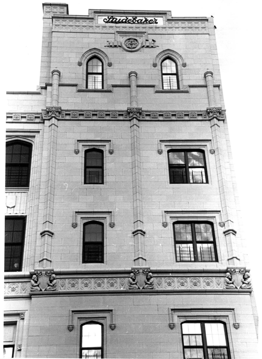
Studebaker Building, detail of tower Photo: Carl Forster
