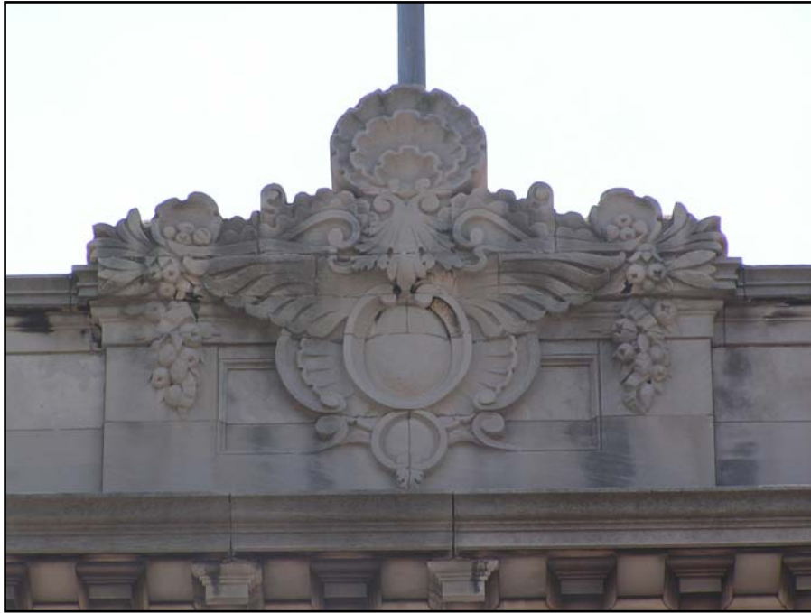
(Former) Jamaica Savings Bank, main façade parapet detail Photo: Michael Caratzas, 2007
