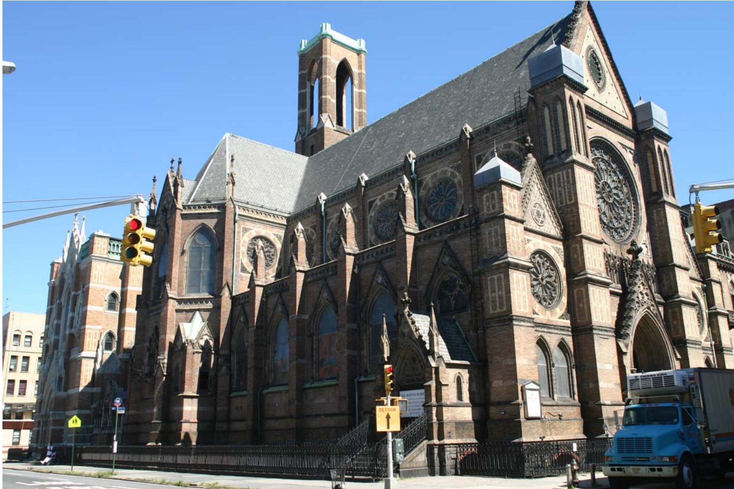
Church of All Saints (Roman Catholic), Parish House and School 47 East 129th Street (aka 50-52 East 130th Street, 2041-2053 Madison Avenue, 41-45 East 129th Street) Landmark Site: Borough of Manhattan Tax Map Block 1754, Lots 20 and 24 Graphic Source: NYC Dept. of City Planning, MapPLUTO, Edition 03C, December 2003
