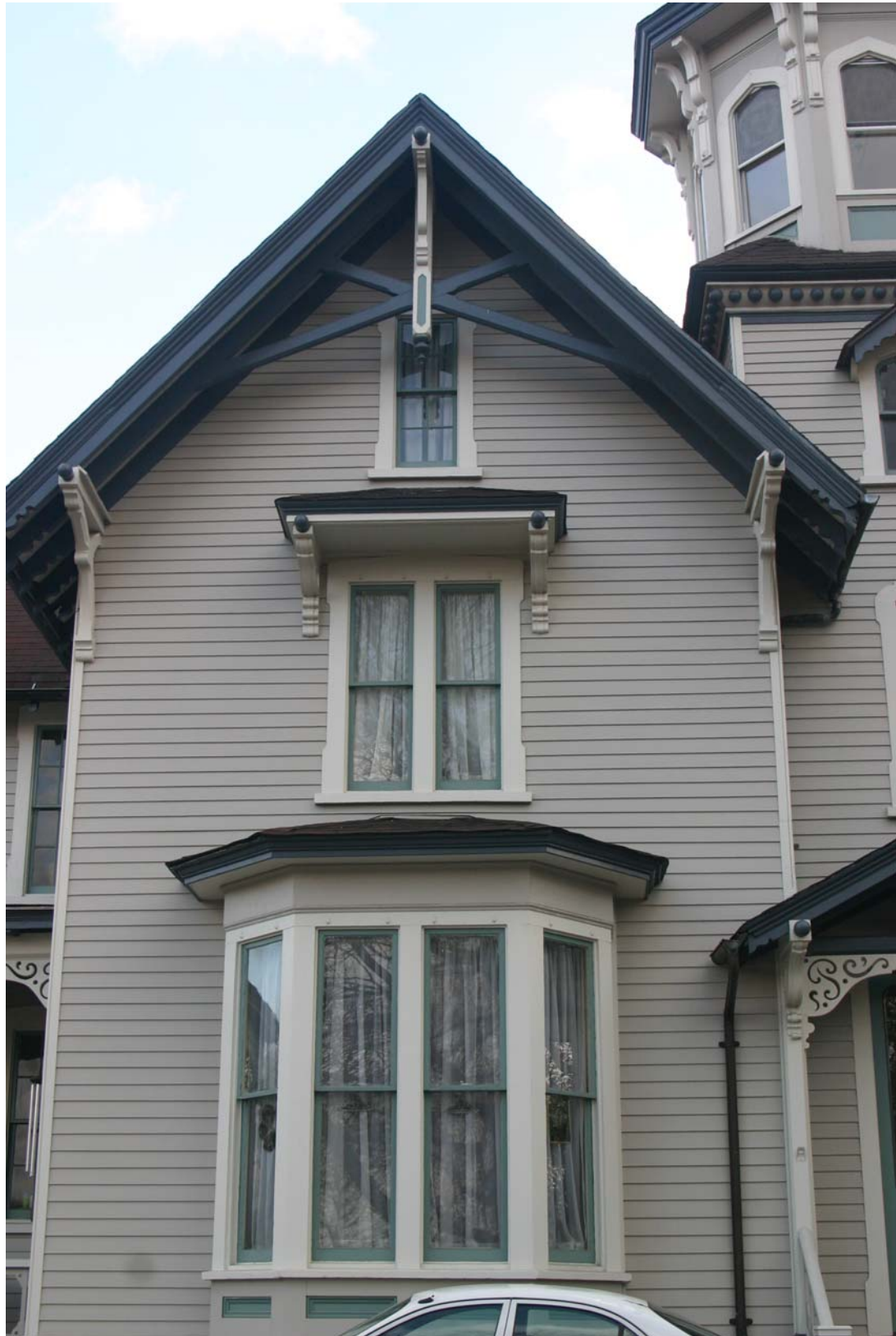
1 Pendleton Place House , gabled bay, north façade Photo, Carl Forster
