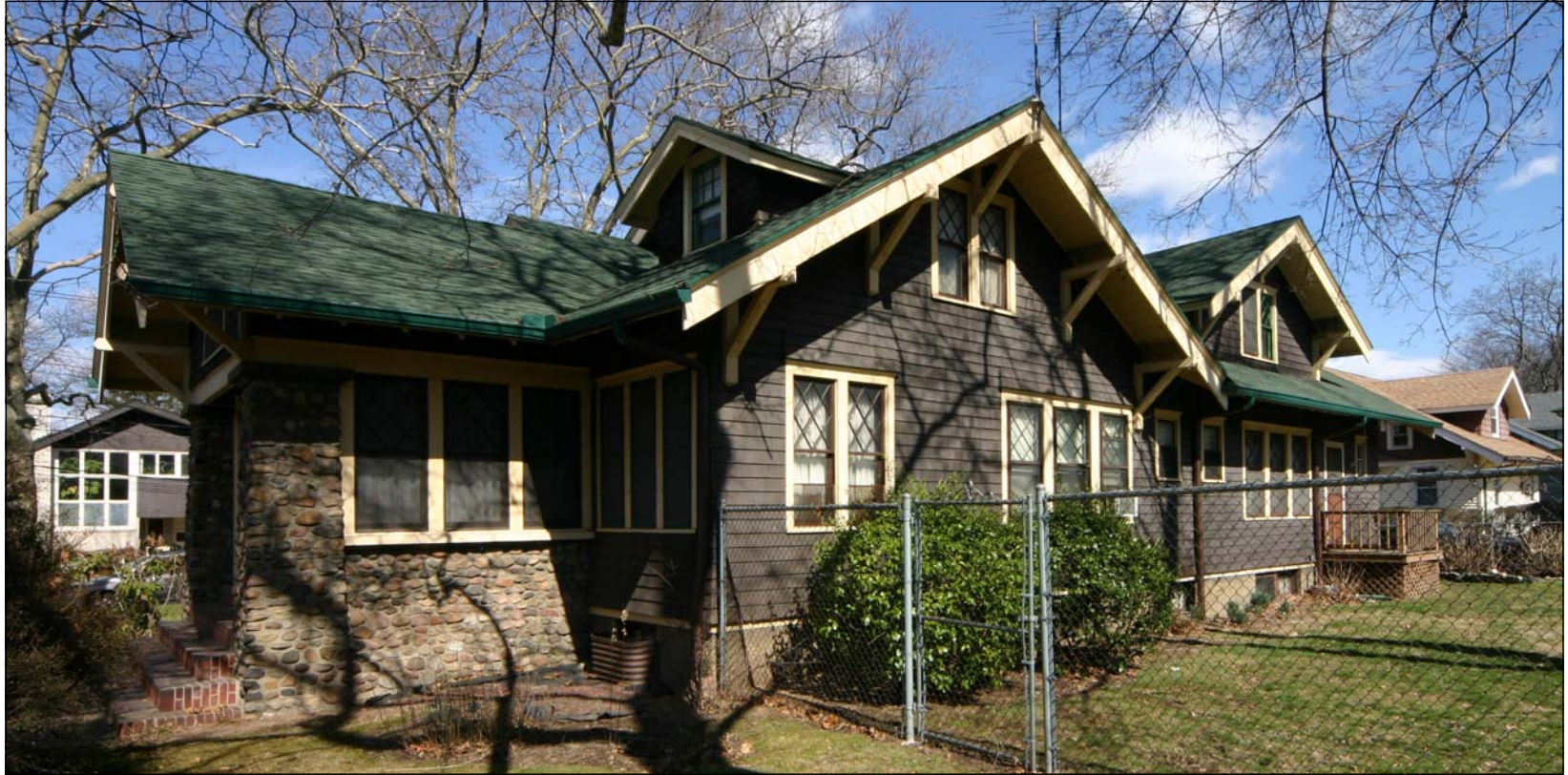
Mark W. Allen House South Façade Photo: Carl Forster
