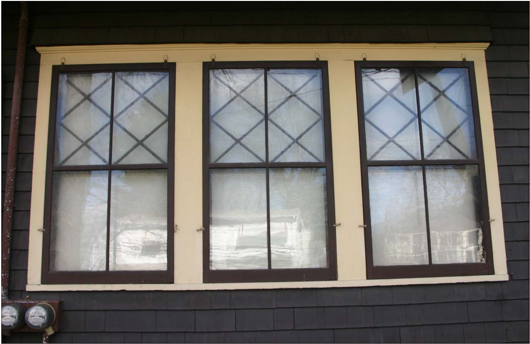
Mark W. Allen House South Façade Detail Photo: Carl Forster
