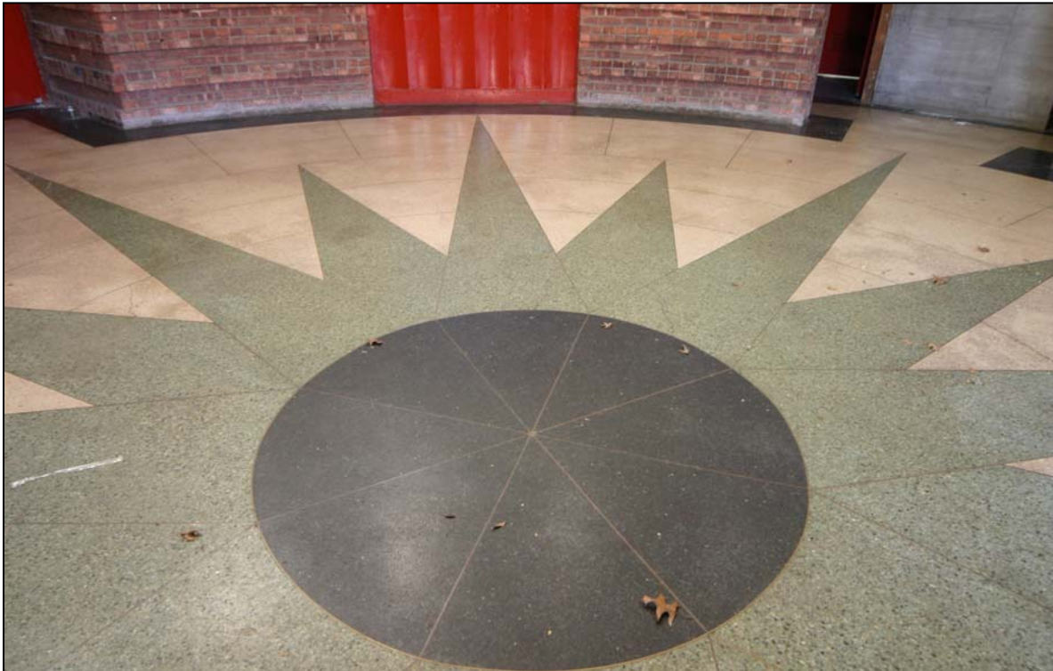
Tompkinsville (Joseph H. Lyons) Pool Bath House Interior: Terrazzo Floor, Lobby Photo: Carl Forster, 2007
