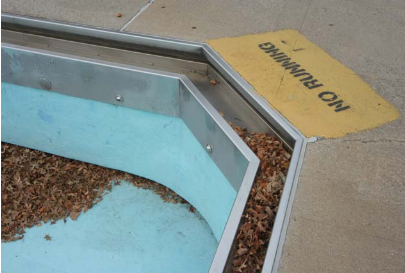
Red Hook Play Center (Sol Goldman Pool): Stainless steel scum gutter, swimming pool Photo: Christopher D. Brazee, 2008
