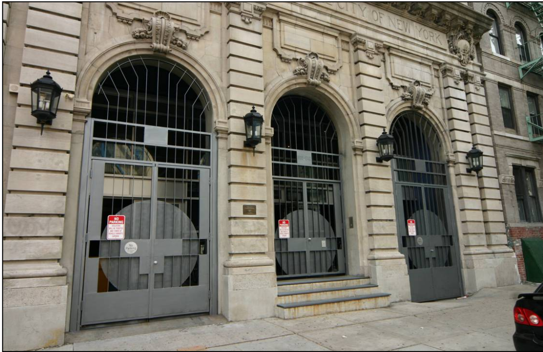
Free Public Baths of the City of New York, East 11 th Street Bath Entryways Photo: Carl Forster
