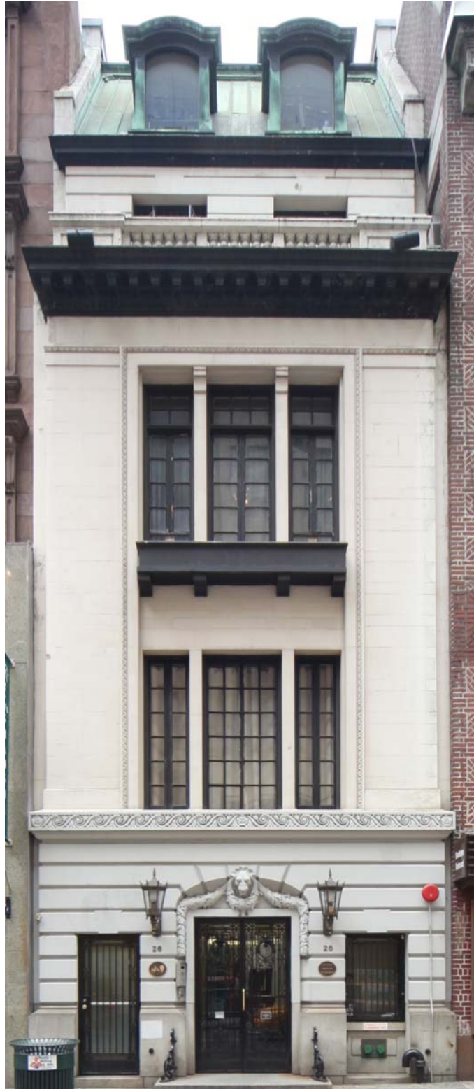
E. Hayward and Amelia Parsons Ferry House 26 West 56th Street, Manhattan Photo: Christopher D. Brazeo, 2009
