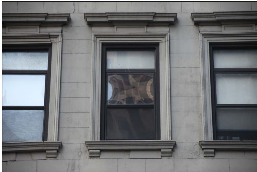
311 Broadway Details of the cornice, quoins and window surrounds Photo: Christopher D. Brazee, 2010
