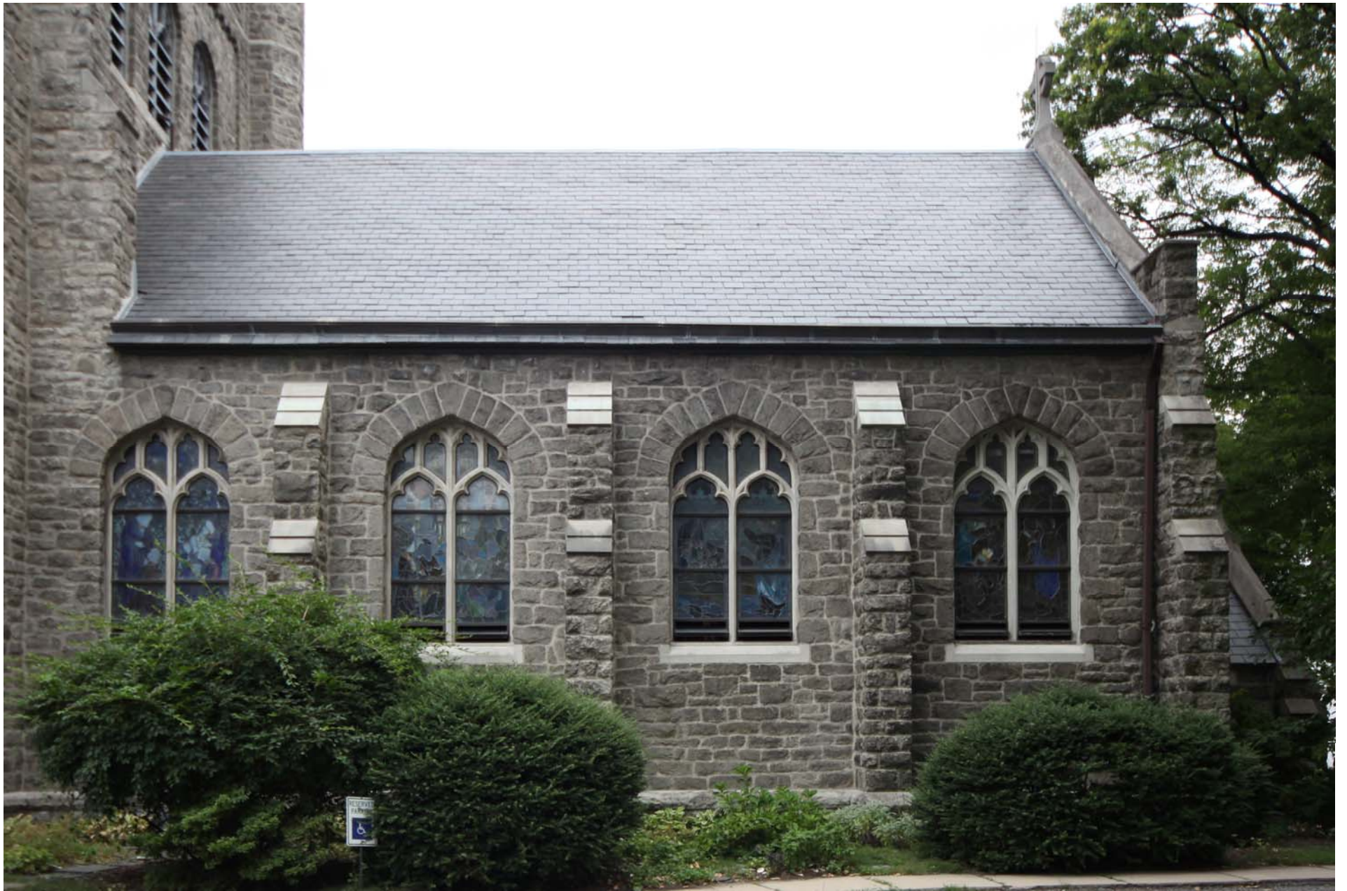
Christ Church South nave wall
