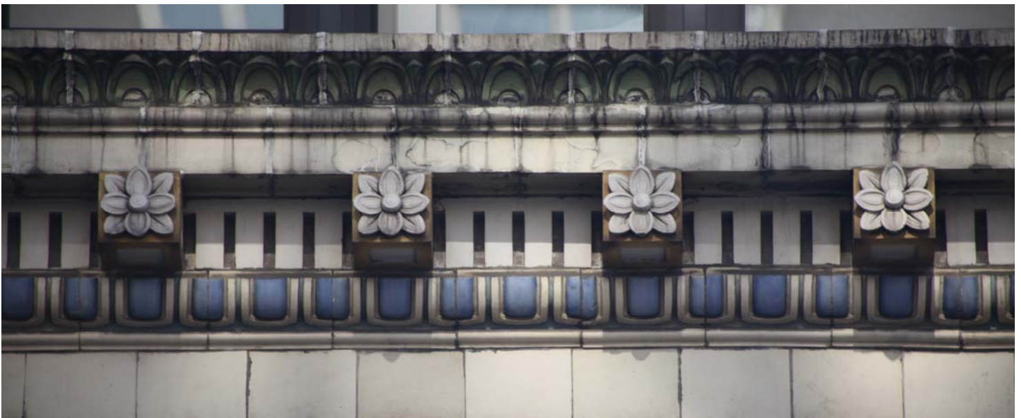
154 West 14th Street Building, terra-cotta details: midsection spandrel (upper) and cornice of base (lower)
