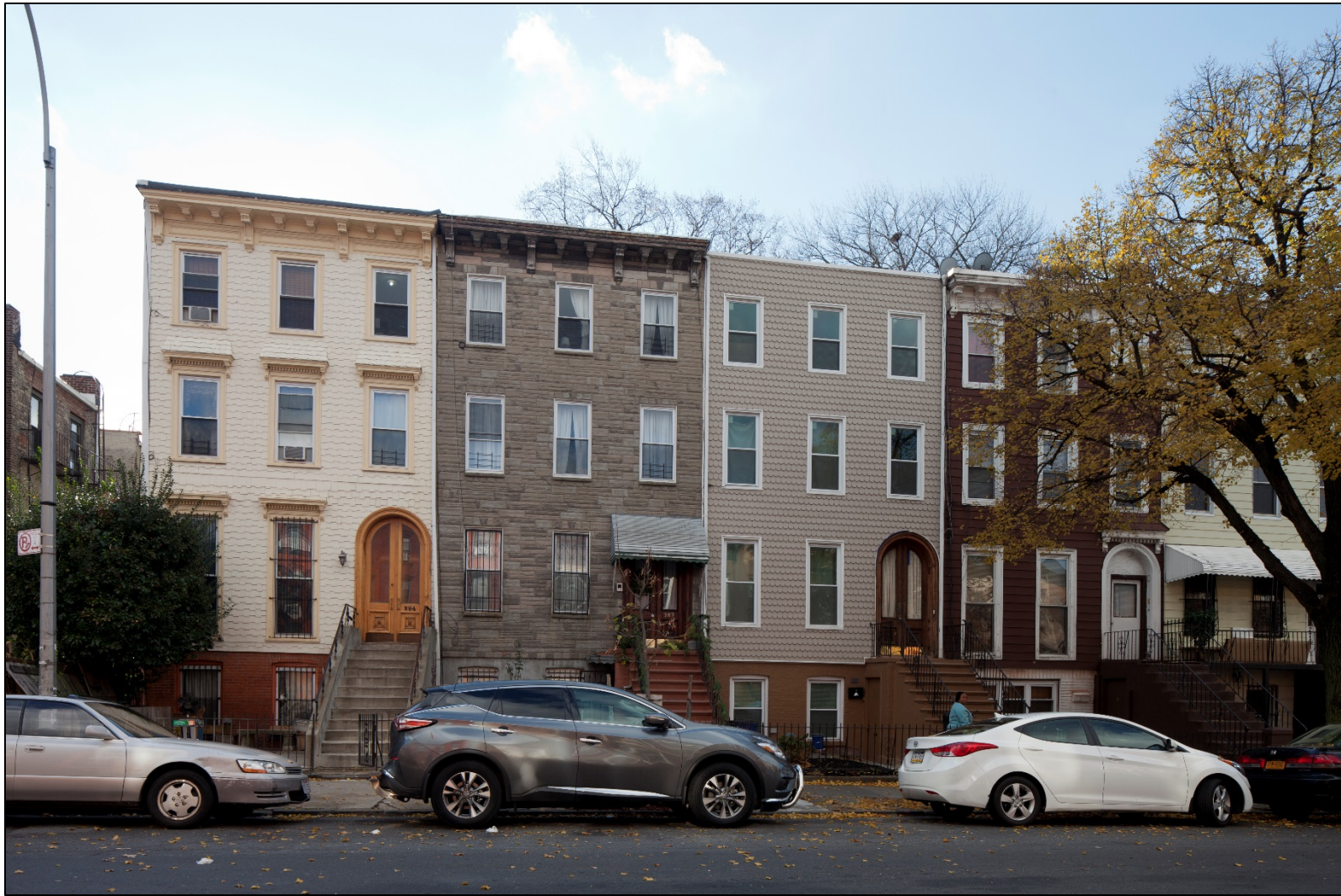
Figure 1 276 to 284 Monroe Street (Walter C. and Susanna E. C. Russell, Developers, c. 1871) Photo: Christopher D. Brazee, 2015
