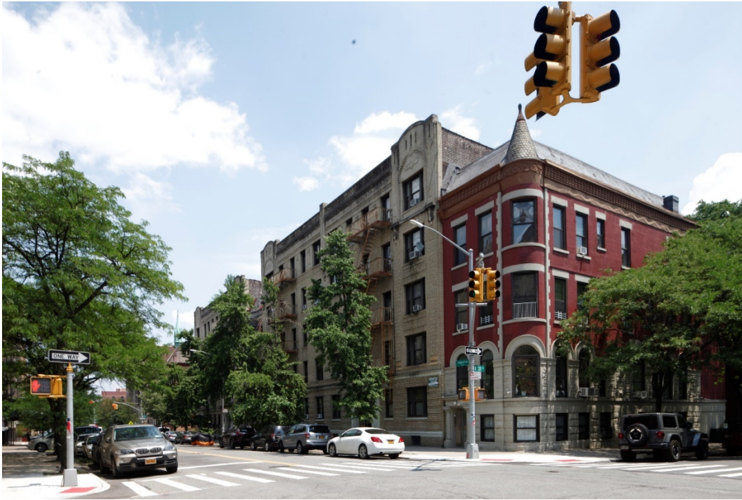
Figure 9 80 Edgecombe Avenue (aka 78-86 Edgecombe Avenue) Jessica Baldwin, LPC, 2021
