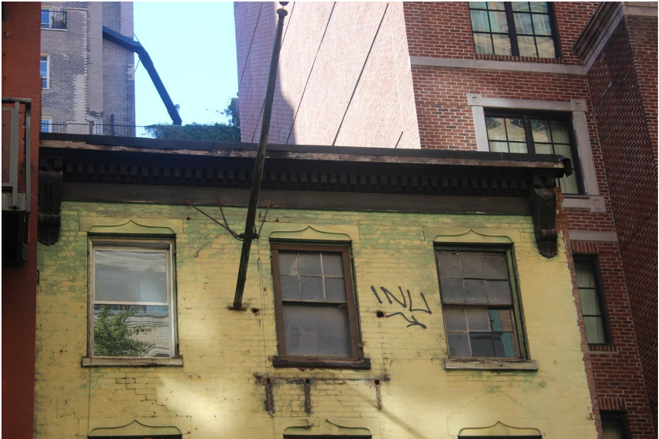
Cornice Detail Sarah Eccles, October 2024
