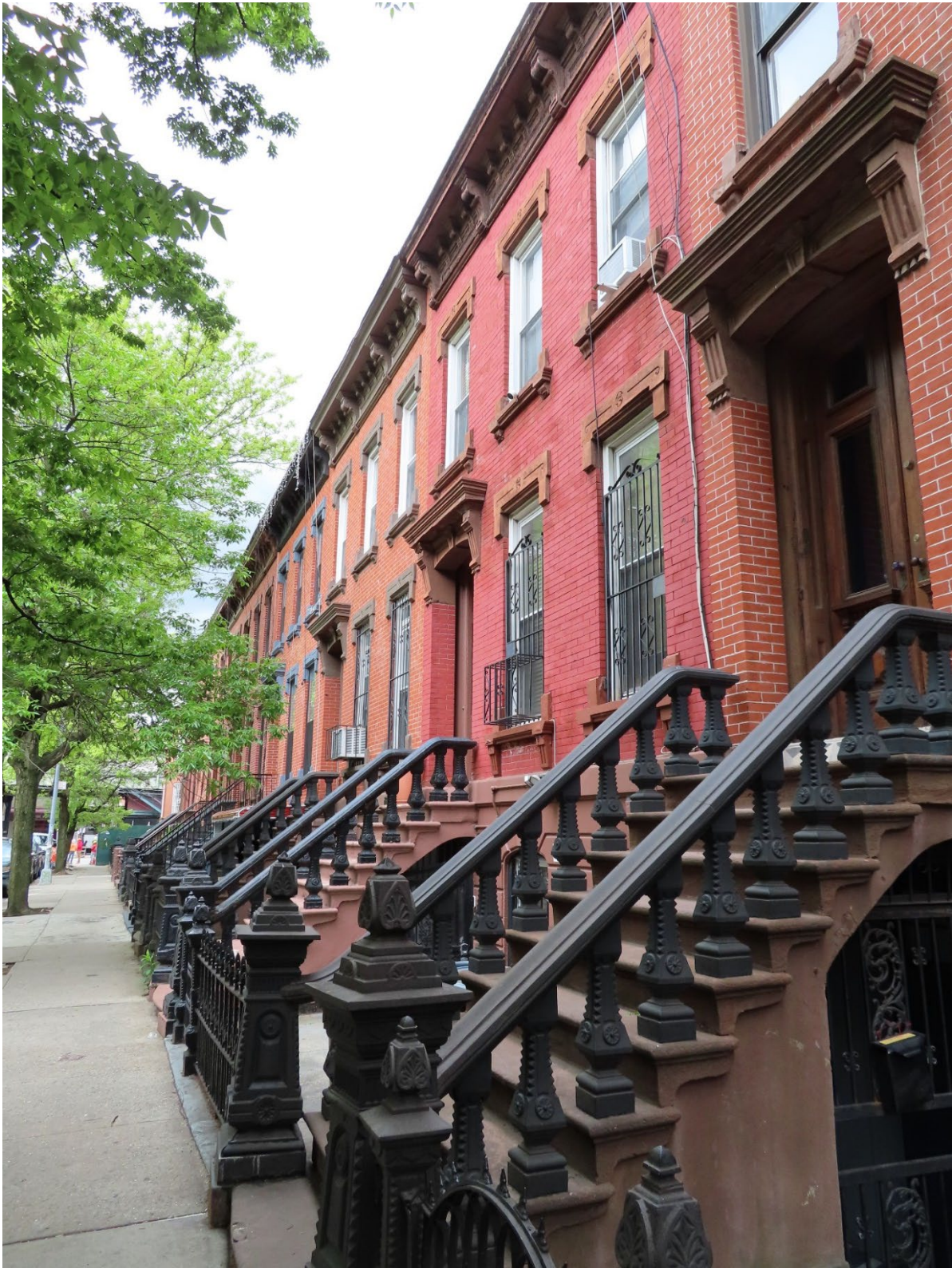
View Toward Broadway along Northwest Side 15 to 35 Linden Street LPC Research Staff, May 2023
