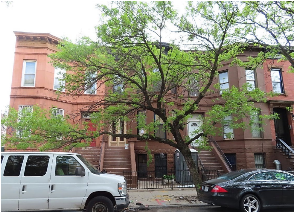
Northwest Side, 15 to 19 Linden Street LPC Research Staff, May 2023
