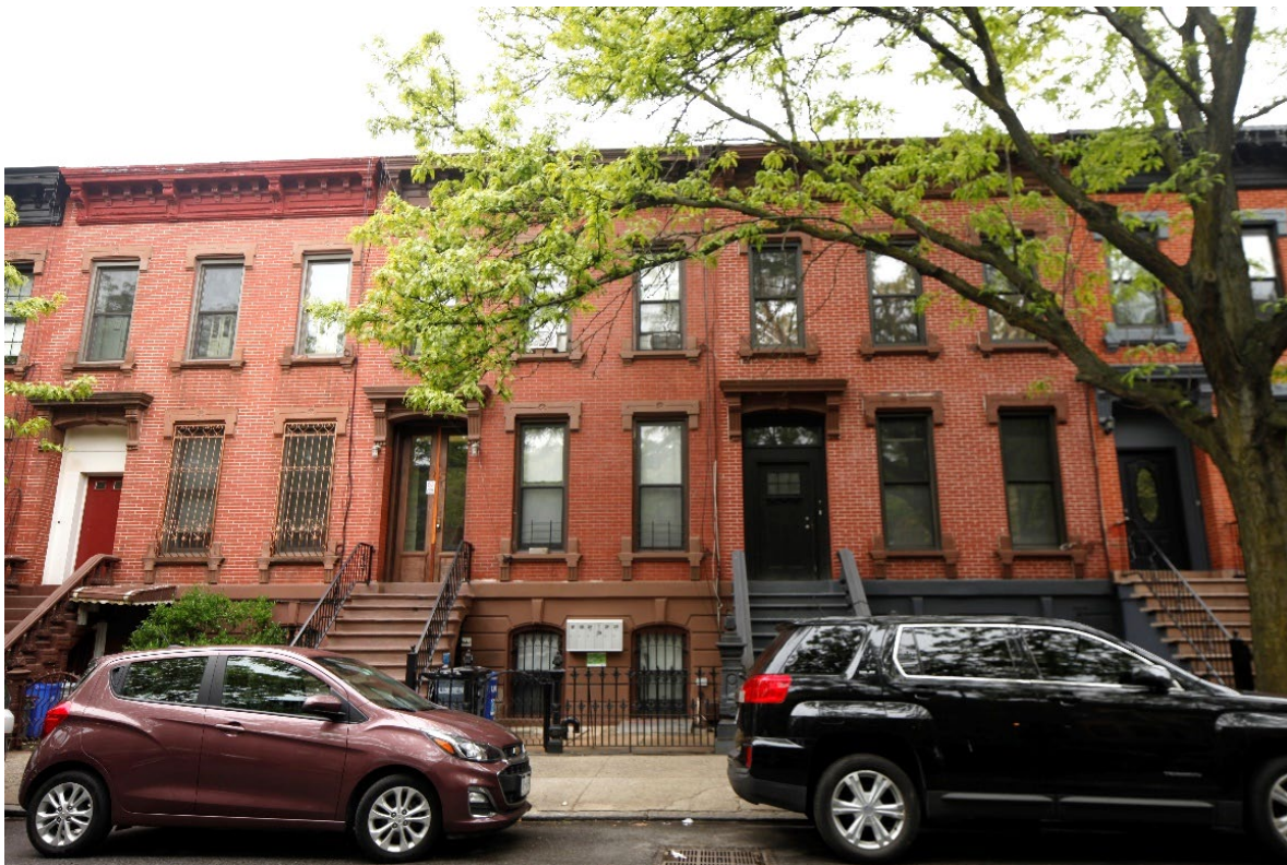
Northwest Side, 23 to 29 Linden Street LPC Research Staff, May 2023
