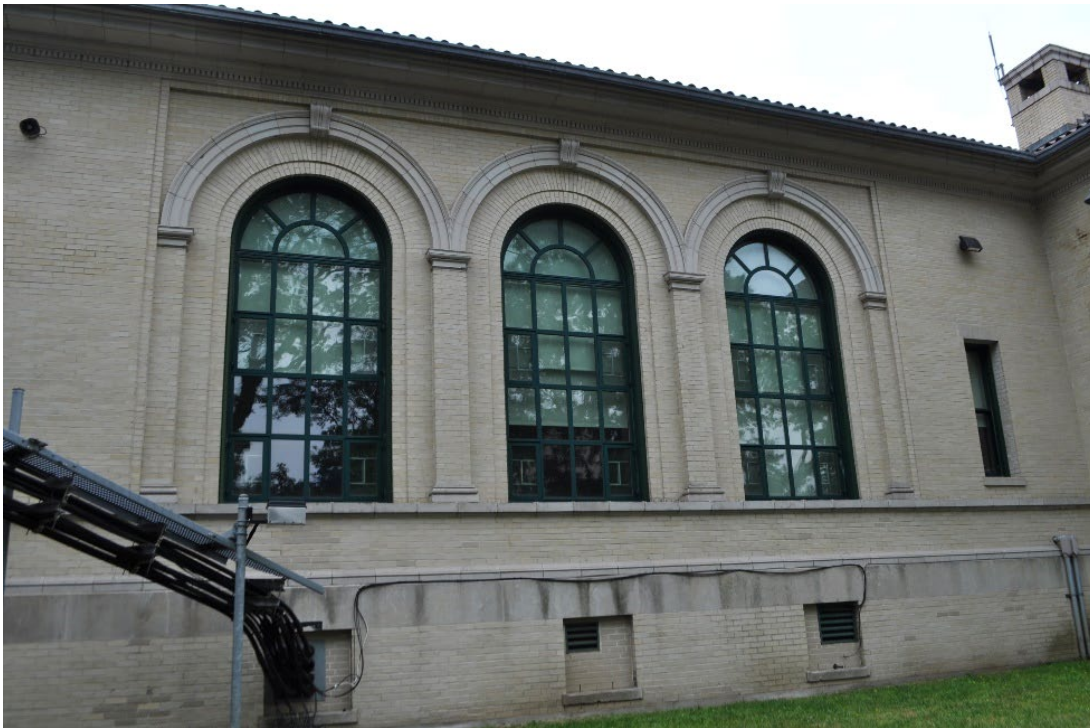
Fire Alarm Telegraph Bureau, Bronx Central Office – Window detail Lisa Buckley, June 2023
