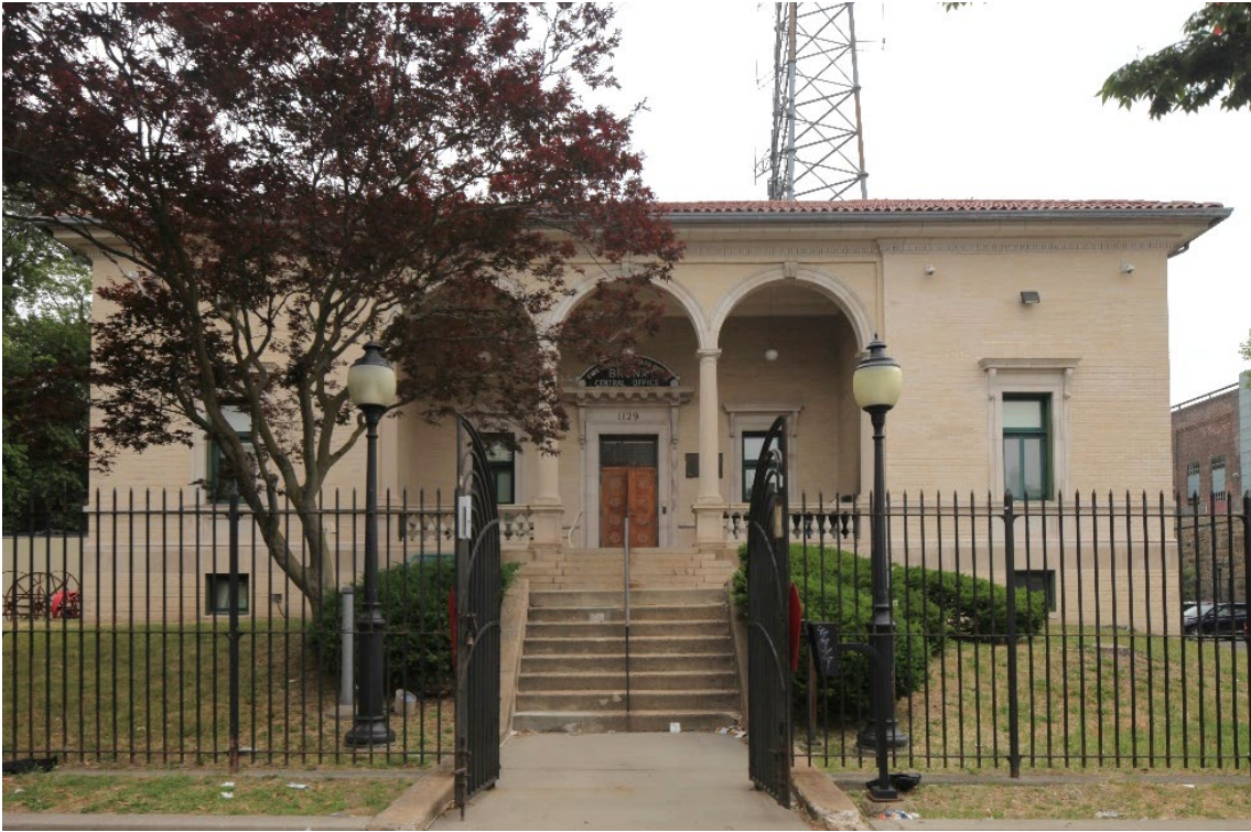
Fire Alarm Telegraph Bureau, Bronx Central Office – South Elevation Bilge Kose, June 2023
