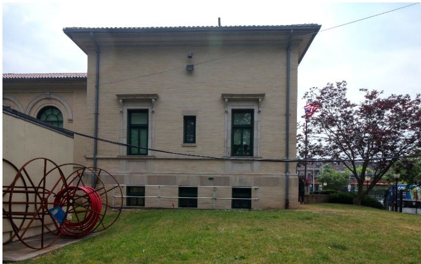
West Elevation, Front Pavilion Bilge Kose, June 2023
