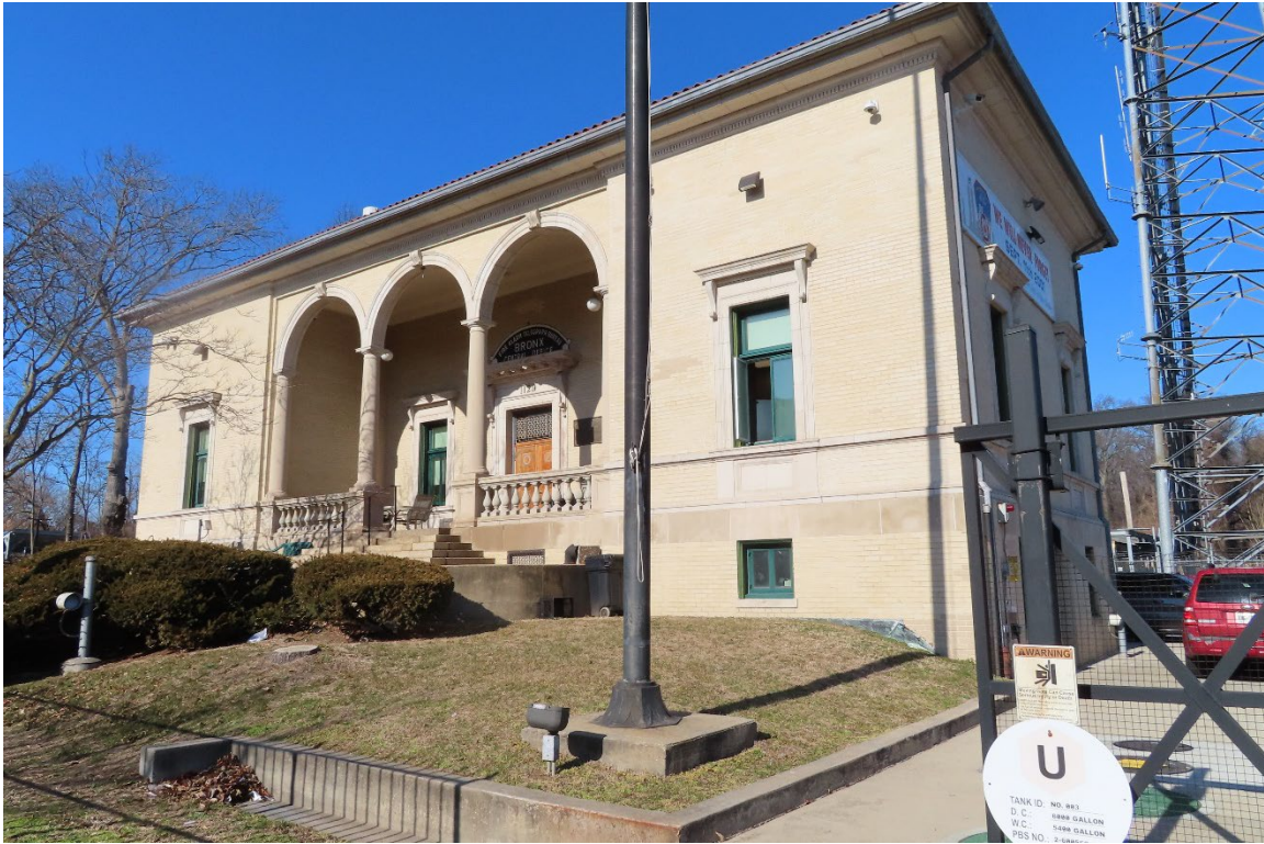
Fire Alarm Telegraph Bureau Michael Caratzas, February 2023
