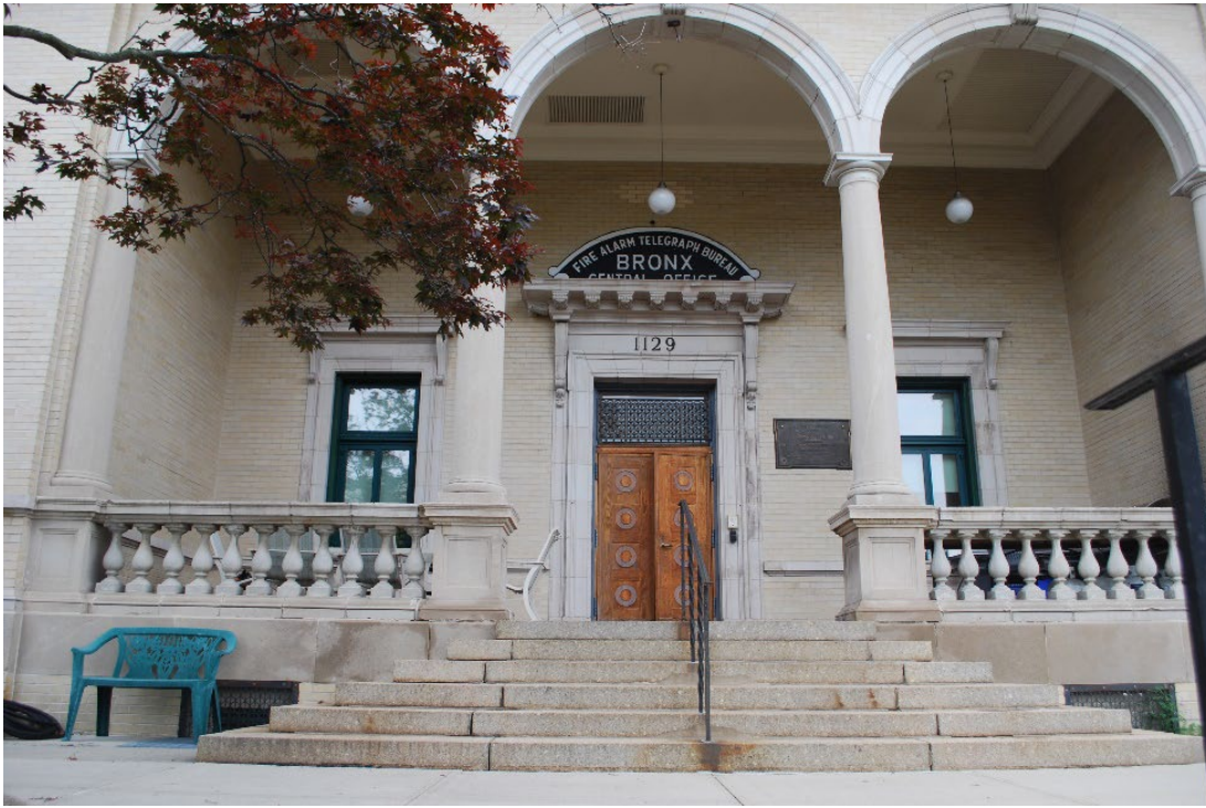
Fire Alarm Telegraph Bureau, Bronx Central Office – Loggia Marianne S. Percival, June 2023
