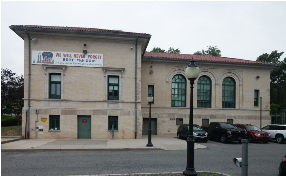
Fire Alarm Telegraph Bureau, Bronx Central Office – East Elevation Bilge Kose, June 2023
