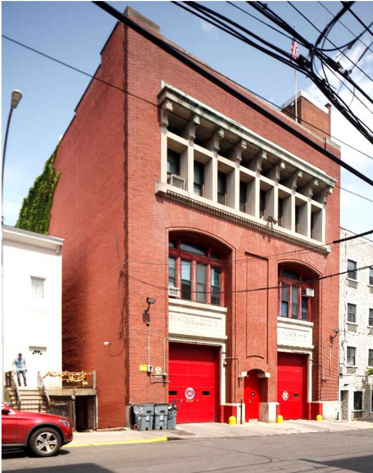
Firehouse, Engine Company 88/ Ladder Company 38 front facade, 2225 Belmont Avenue, Bronx Lisa Buckley, June 2023
