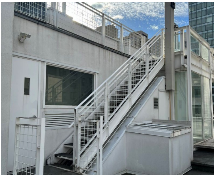
Roof deck stairs LPC, December 2023
