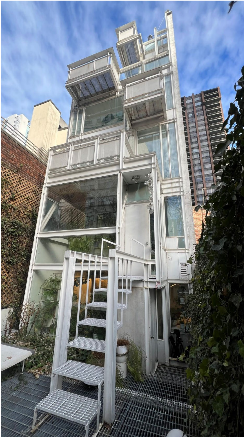
Modulator Building, rear facade LPC, December 2023
