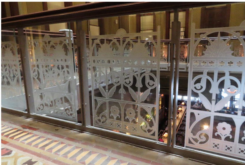
Second story gallery balustrade detail Marianne S. Percival, May 2024
