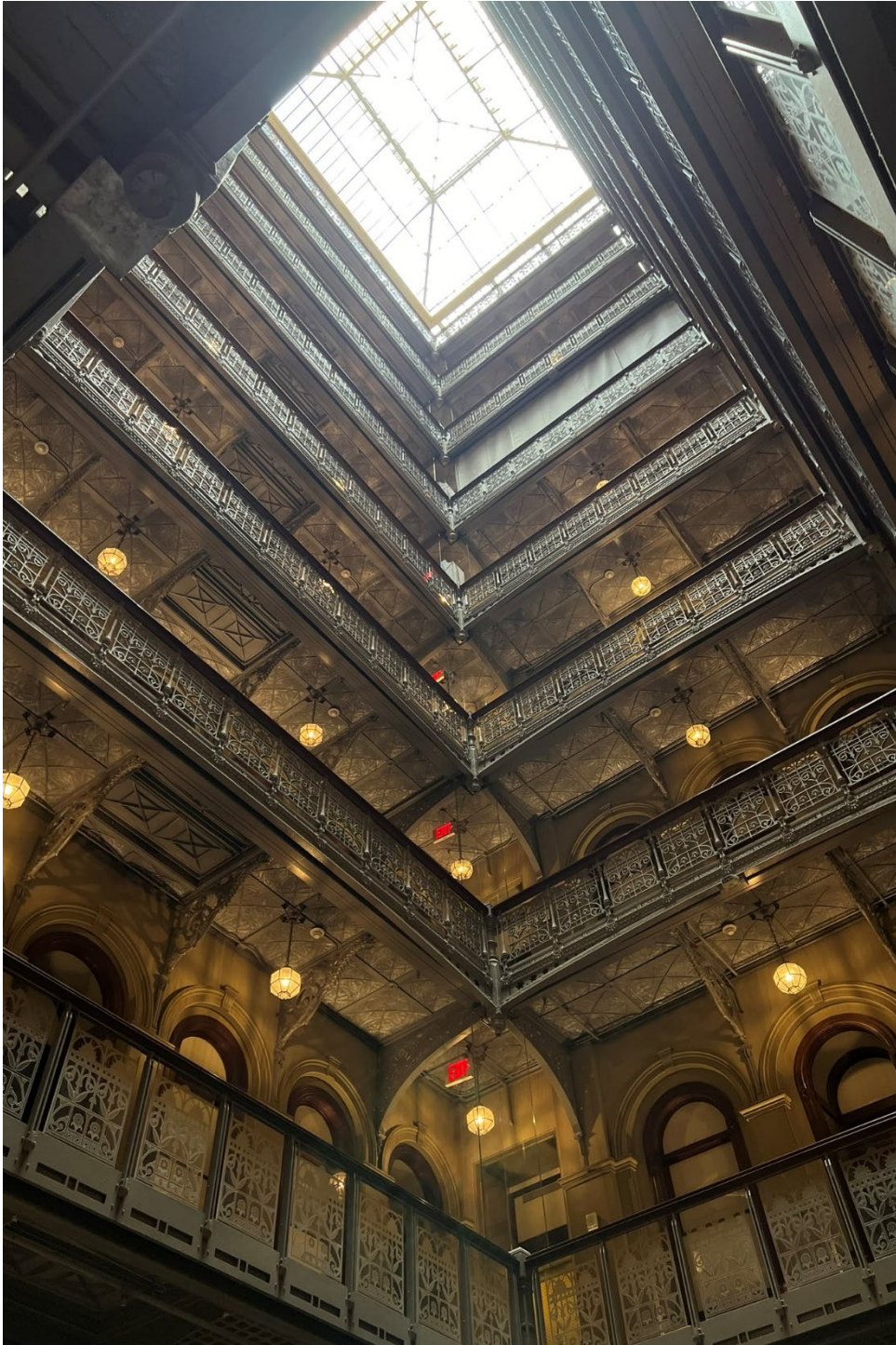
Temple Court Building (now The Beekman Hotel) Atrium 5 Beekman Street (aka 3-9 Beekman Street; 119-133 Nassau Street; 10 Theatre Alley) Bilge Kose, May 2024
