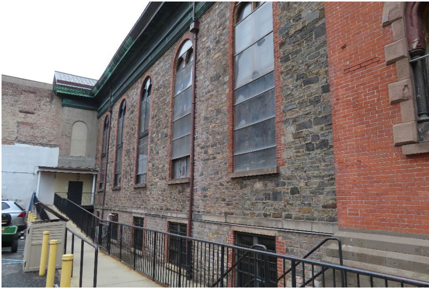
West Facade Lisa Buckley, April 2026
